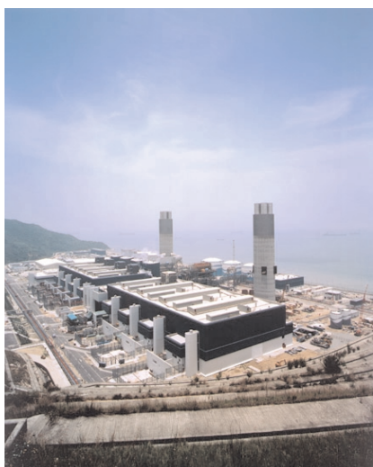
Figure 46. Indoor S109FA installation
